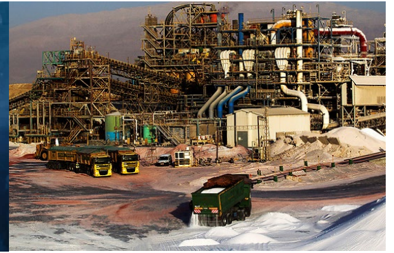
Preventative Maintenance Inspection
